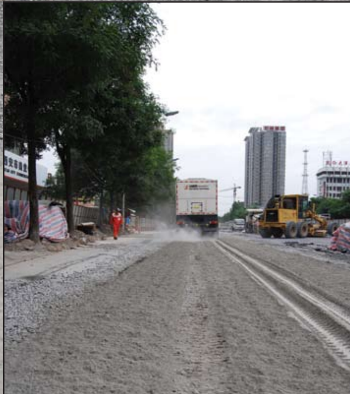
Spreading the remaining width of 0.82m
