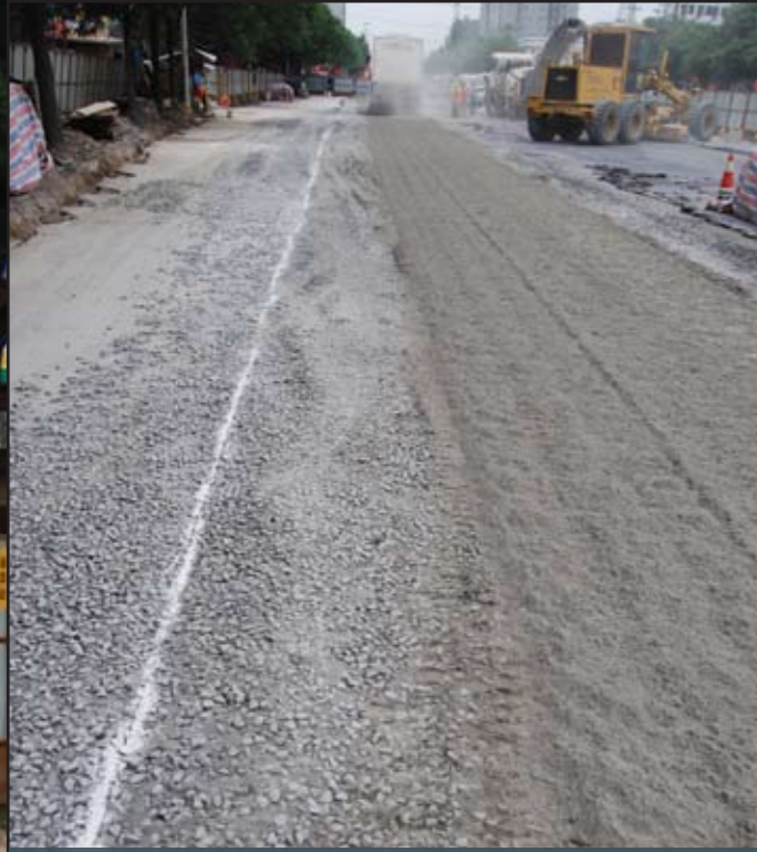
Spreading a width of 2.46 m
