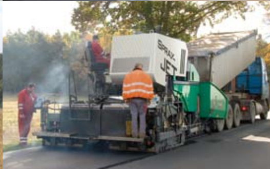
The SUPER 1800-2 with SprayJet Module handles all your resurfacing contracts in a highly efficient, economical and clean manner.
